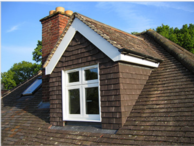
Gable dormer window
