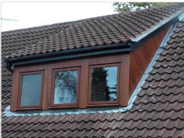
Catslide dormer extension
